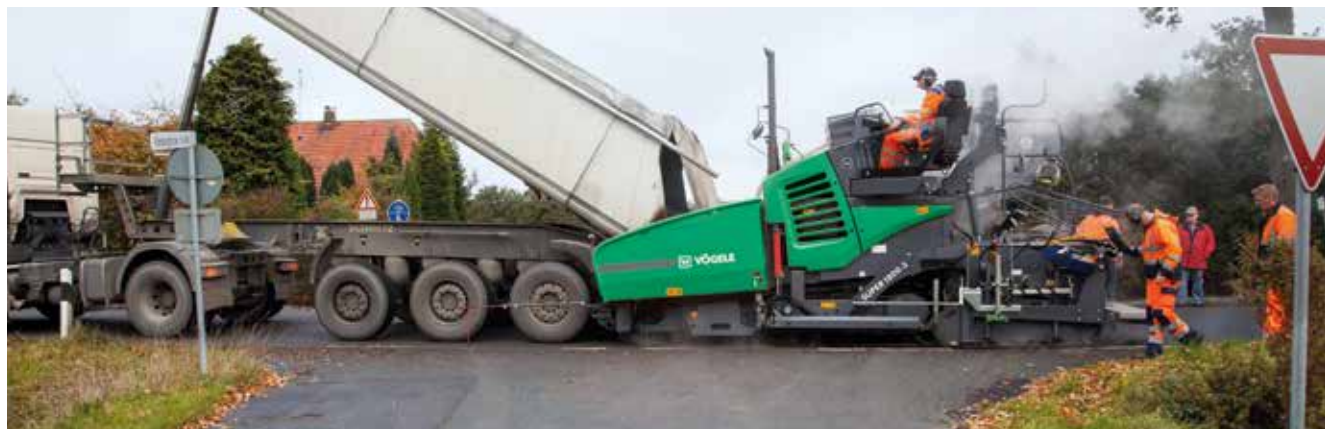
RESURFACING A ROADWAY IN A RESIDENTIAL AREA
