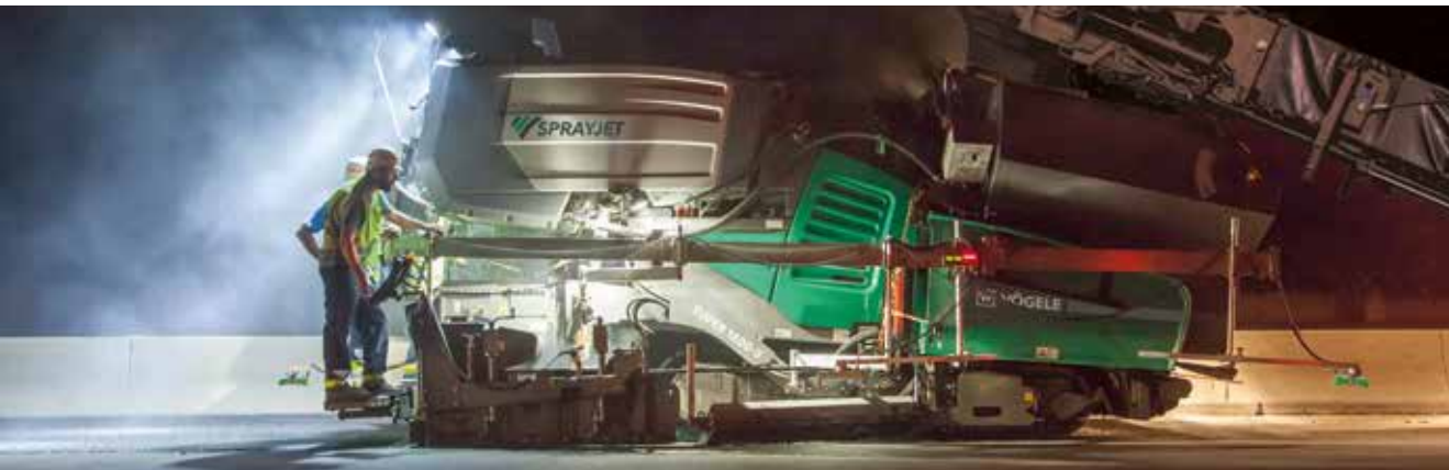
RESURFACING WORK ON A MOTORWAY
